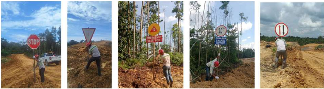
Gambar 8. Pemasangan Rambu Jalan di Area Kerja WMP 04 GT ( Control Traffic Management )
